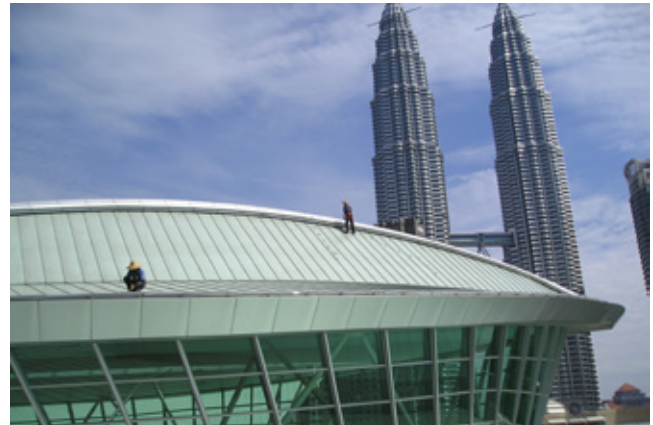
Kuala Lumpur Convention Centre, Malaysia
