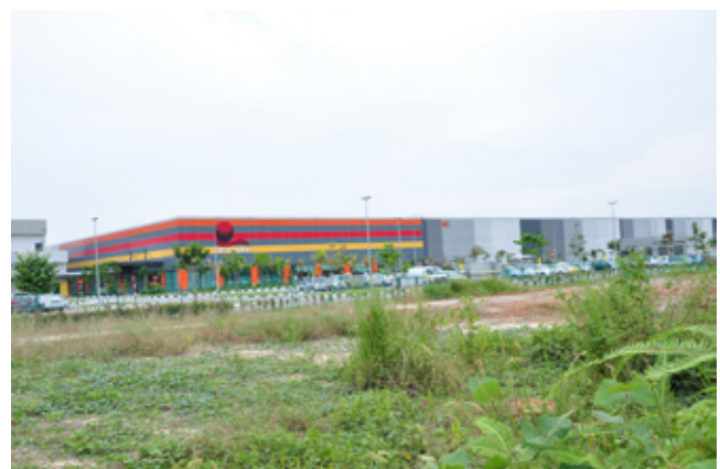
First Solar photovoltaic plant, Kulim, Malaysia
